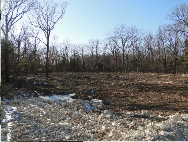
Removal of Trees and Site Leveling
